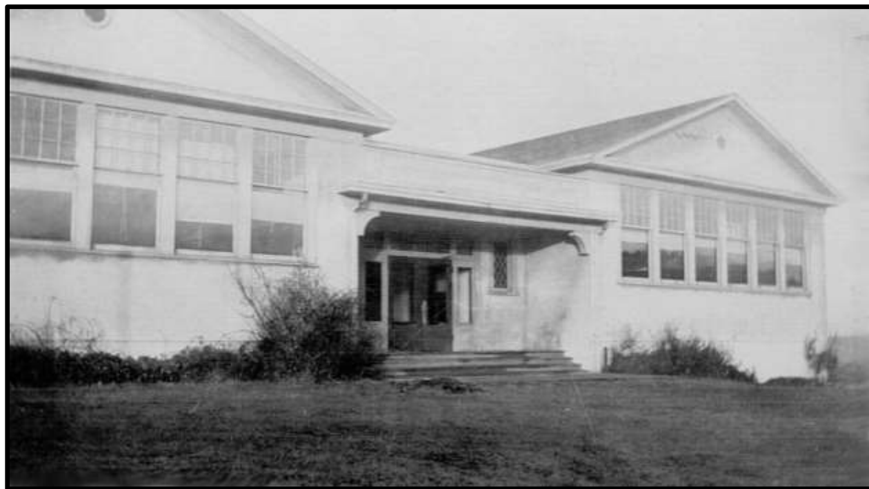
Photo shows east side entrance to Port Orford High School.
